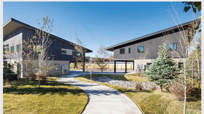
TCSD HOUSING PROJECT
