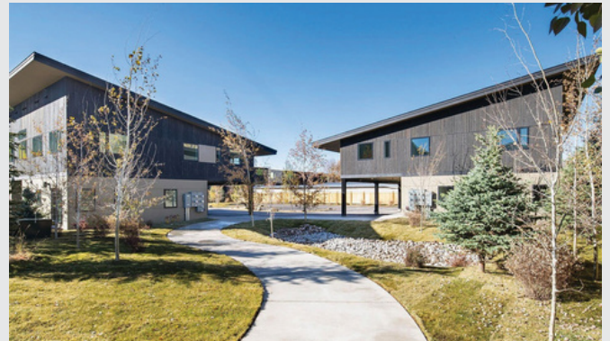
TCSD HOUSING PROJECT
