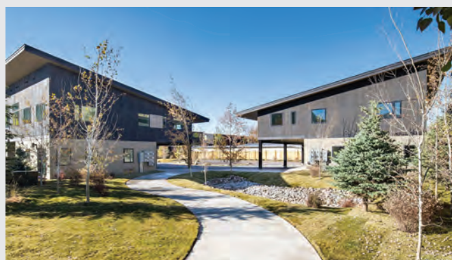
TCSD HOUSING PROJECT
