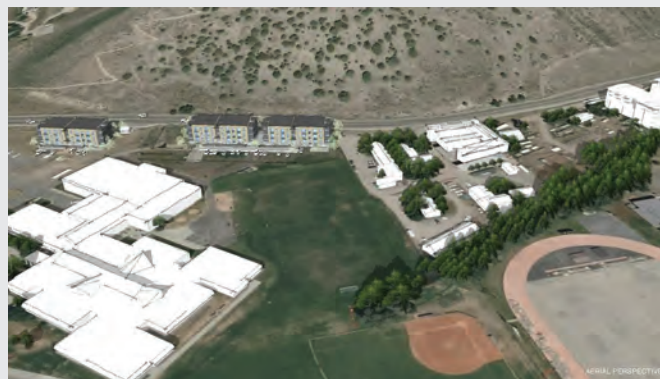
TCSD HOUSING PROJECT
